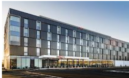
Hotel Ibis, Bridgewater Woodlands Court Business Park, Bristol Road
